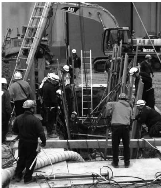
Illinois Fire Service Institute Spring 2014
